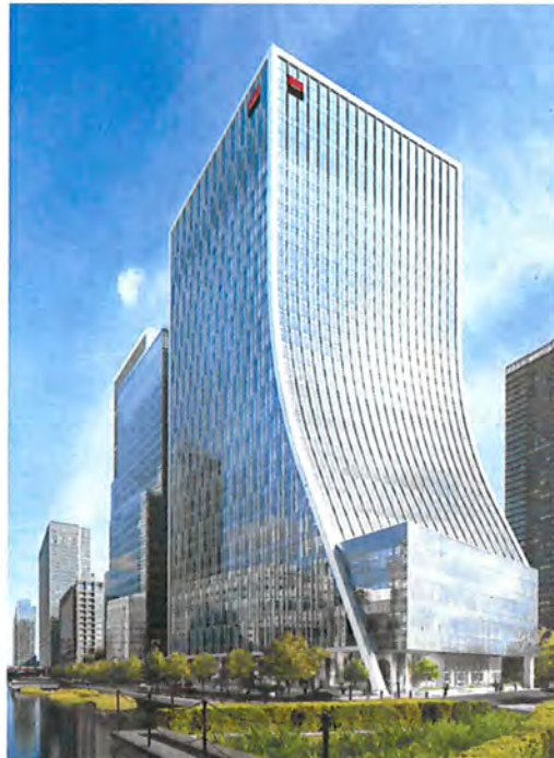
One Bank Street. The SG Canary Wharf Office Building
